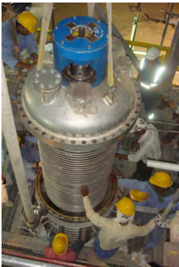
FUNDA Filter Installation
